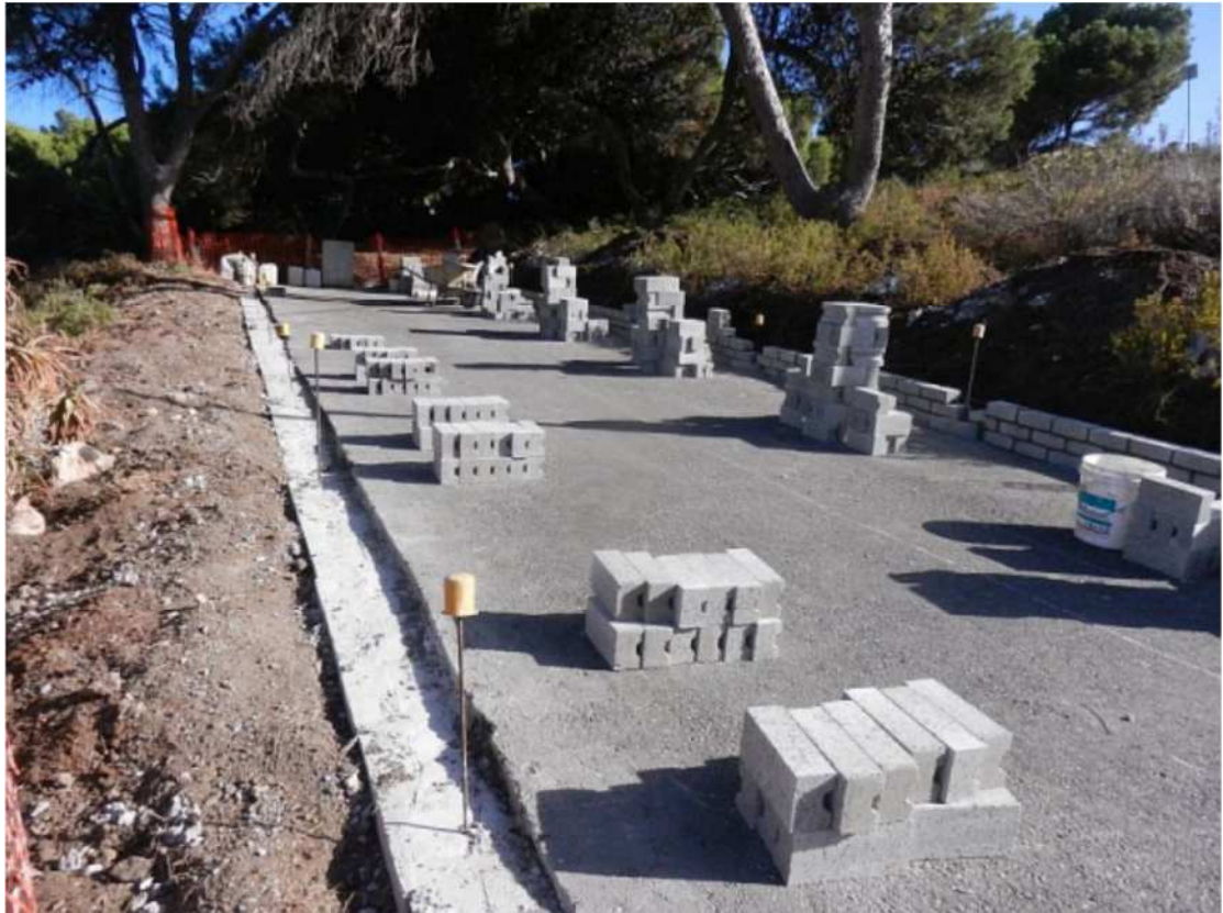
The wall slowly growing.
