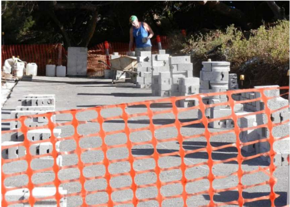
Stone Mason Paul Freebairn commencing work on the wall.
